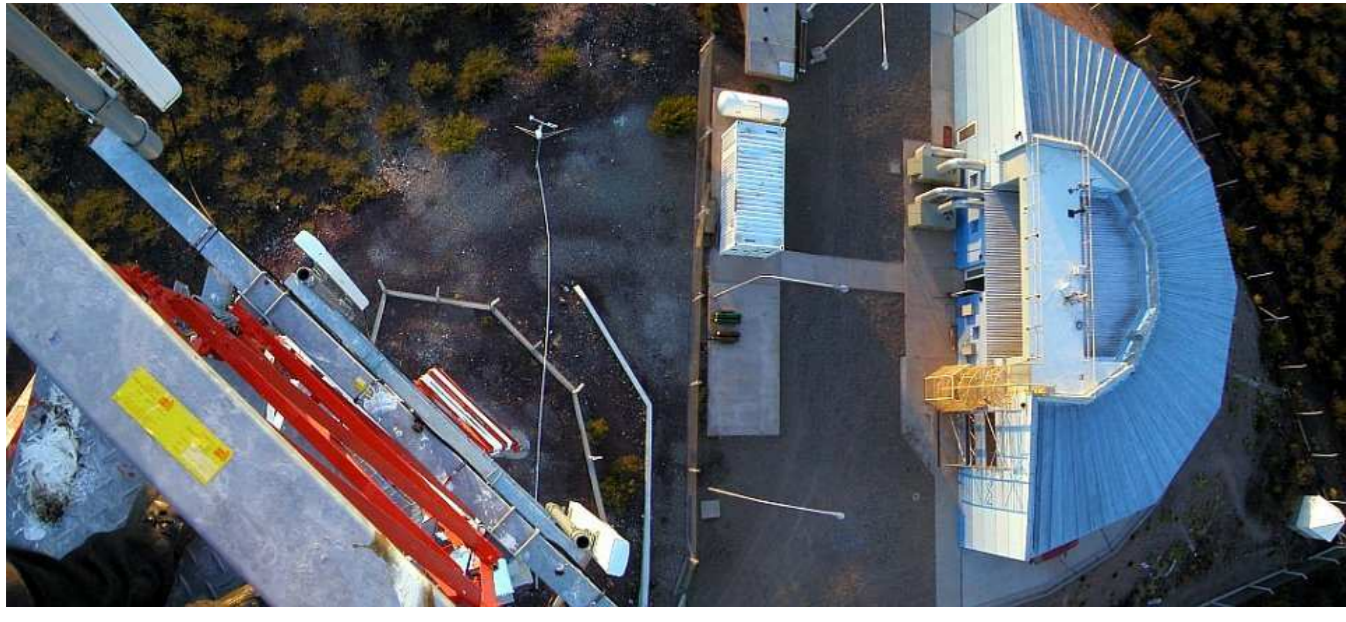
Pierre Auger Observatory is a cosmic-ray detecting facility built and operated by Auger Collaboration near Malargue in Argentina. The observatory consists of two cooperating, but observationally independent detectors: Surface detectors (SD) are water Čerenkov tanks with photomultipliers covering in a regular grid an area of \sim 3000 \text{ km}^2 ; Fluorescence detectors (FD) is a system of 24 segmented 3.6 m telescopes observing fluorescence in the atmosphere above the SDs. The image is taken from the communication tower shows one of four FD Los Leones (containing 6 telescopes), where FRAM is located (small white square in the corner).
