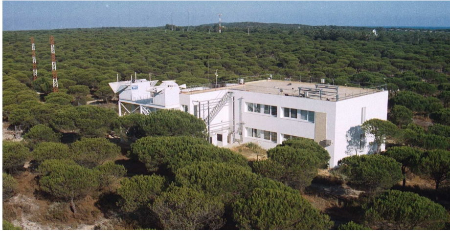
Figure 12: The building of ESAt with domes of BOOTES-1A and BOOTES-1B (2002).
